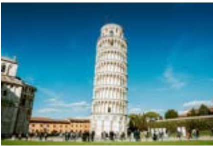
Leaning Tower of Pisa
